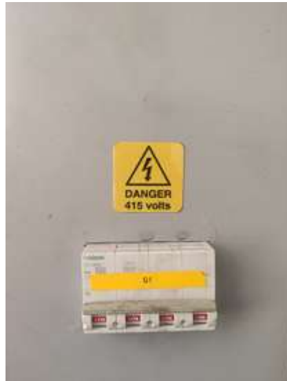
Figure 4-1 Isolator / LOTO switch
