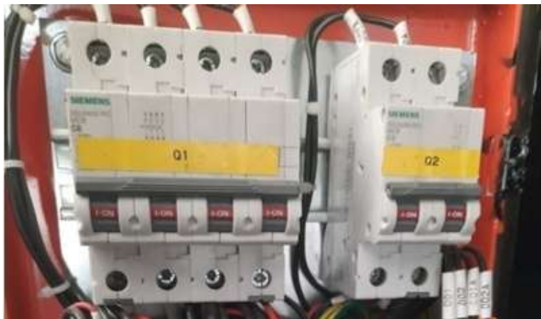
Figure4-1Isolator/LOTO switch
