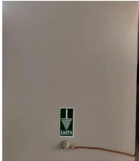
Figure 3-7 PE / Ground connection on Panel and Machine
